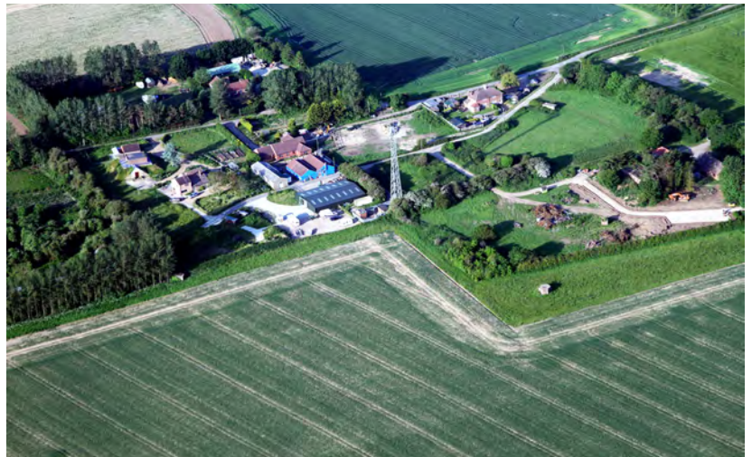
Above West Beckham: The Tx site is just out of picture to the left, the operations centre is the first building on the left still earth covered. The Rx site is on the right with the excavator near the Rx block. Mast is modern – for TV Below left Darsham Radar Rx block visible in the trees. Agriculture reclaimed the rest Below right Bawdsey Manor, home of radar and its initial development
